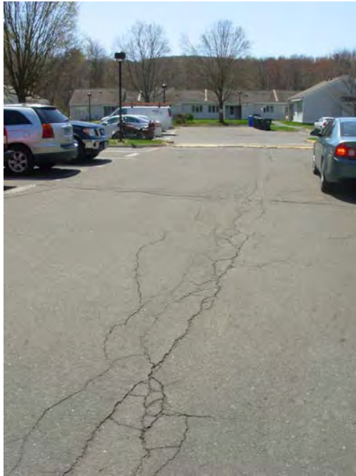
1. Cracking of asphalt paving at parking areas
