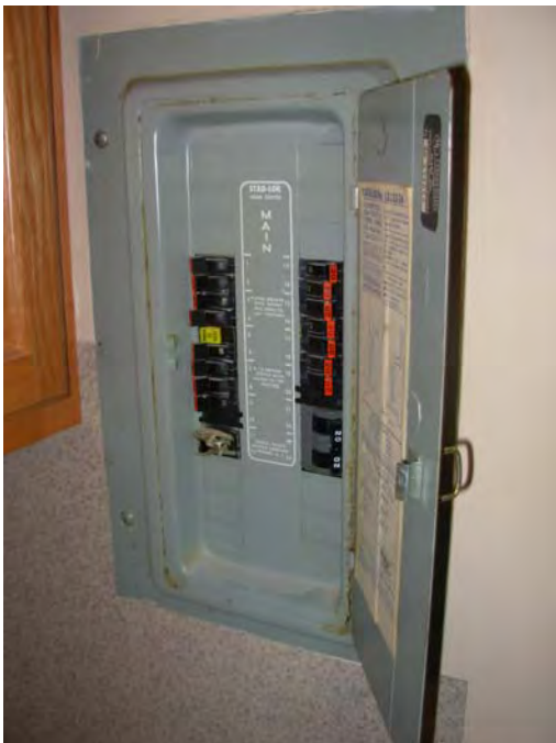
15. Federal Pacific Stab-lok circuit breaker panels, to replace Twenty One • Capital Needs Assessment • © On-Site Insight
