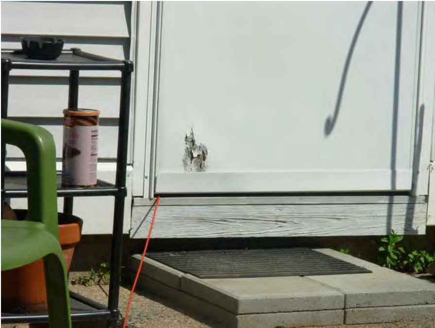
5. Storm door deterioration observed
