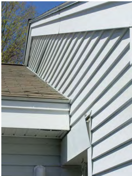
3. Spot siding and trim wrapping damage
