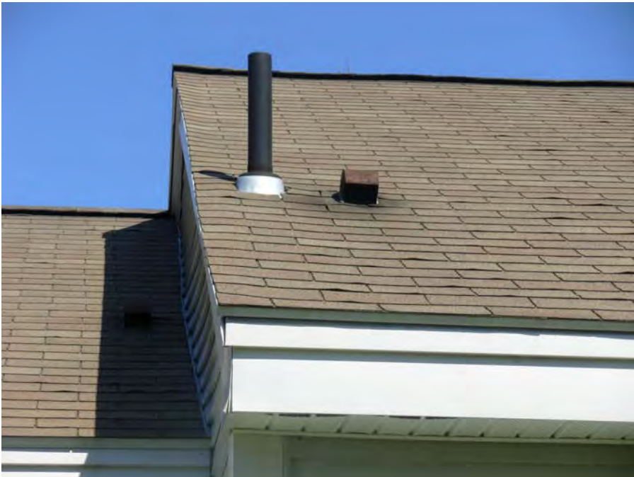
7. Older lifting shingles and decking deflection
